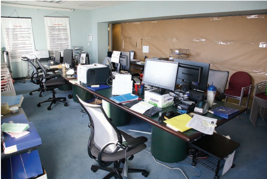
The former Conference room was used as a 'swing space' for various departments and employees who were temporarily relocated pending completion of their new area. A new and larger Conference room is under construction.
