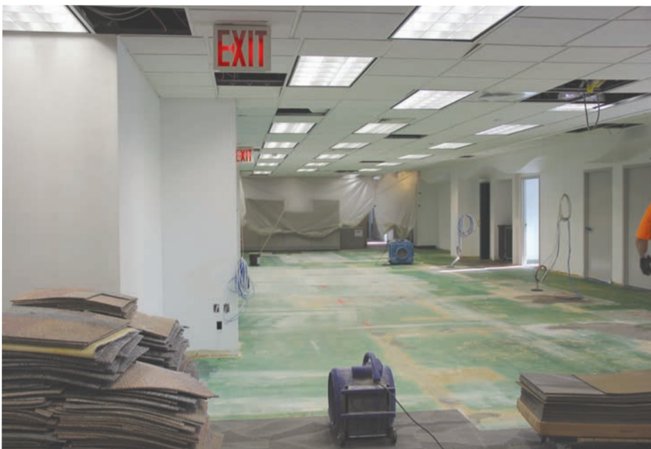
Renovation of the area where the Grapevine workstations will be located.
